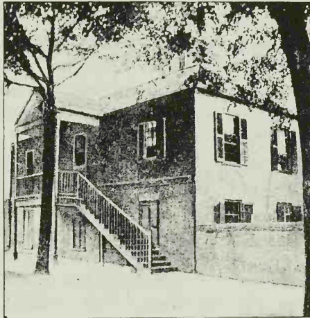
AN OLD MASONIC BUILDING IN WILMINGTON, NORTH CAROLINA
